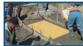
The Paver Unit is pressed flush into wet concrete, tamped in place, and any residual debris is removed from the paver surface.
